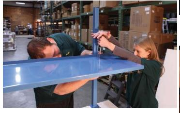
The laminate shelf comes with 4 preinstalled screws. Align the screws with the holes in the shelf brackets.
