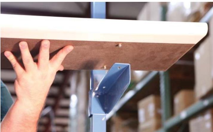
Slide the shelf back into the bracket and tighten the screws.
